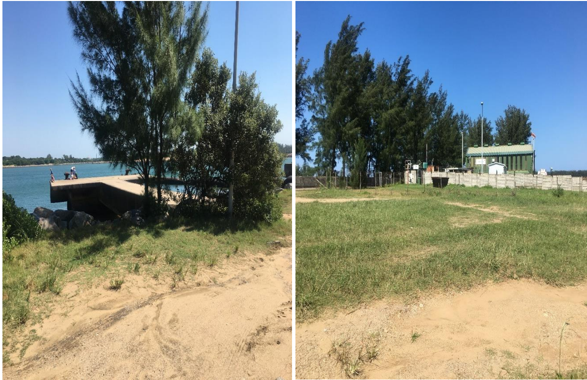
Figure 6: View of structures noted in the area proposed for upgrade.
