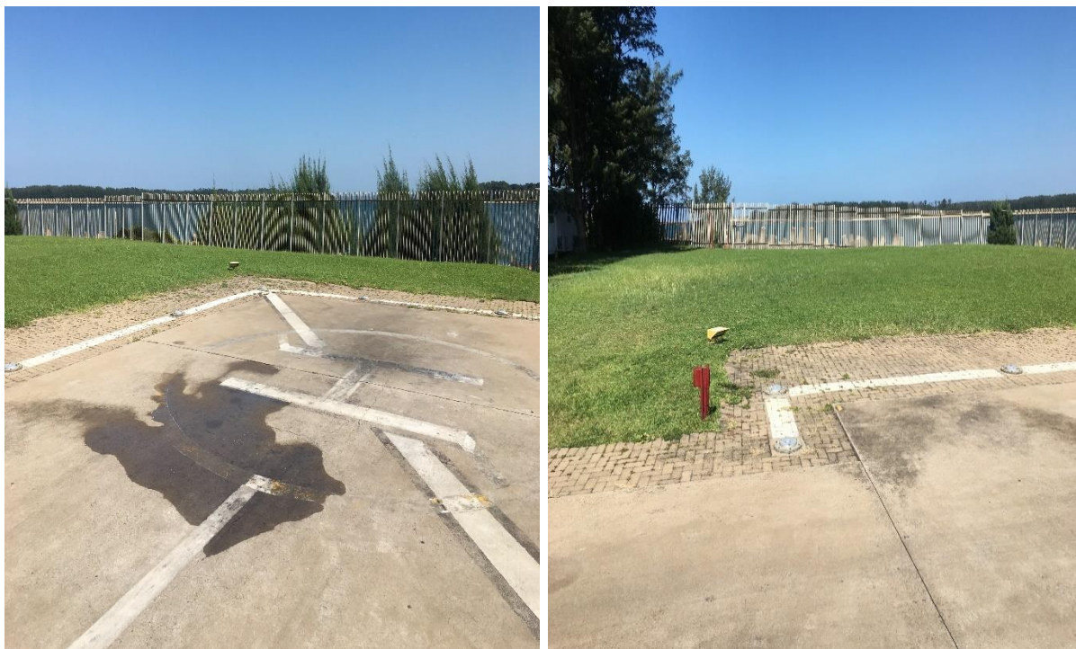
Figure 3: View of the existing helipad proposed for upgrade.
